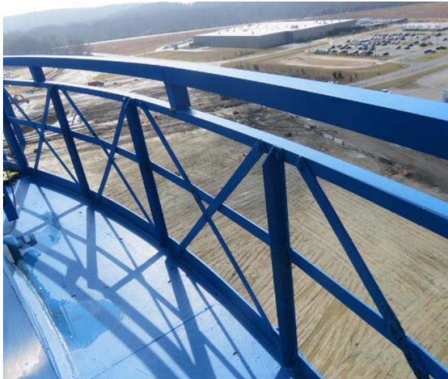
Existing Water Tank Handrail Inside View (Typical)
