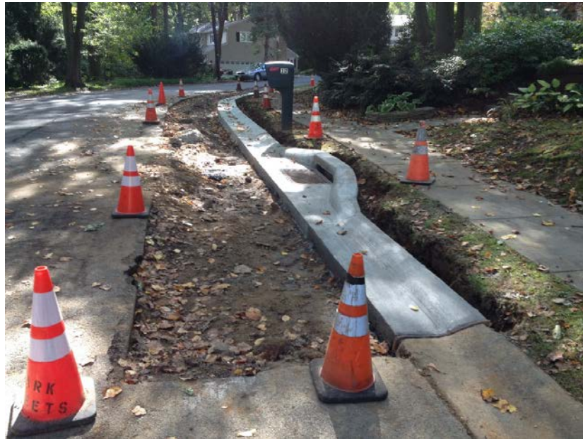
Concrete Curb and Bonnet Repairs at Blue jay
