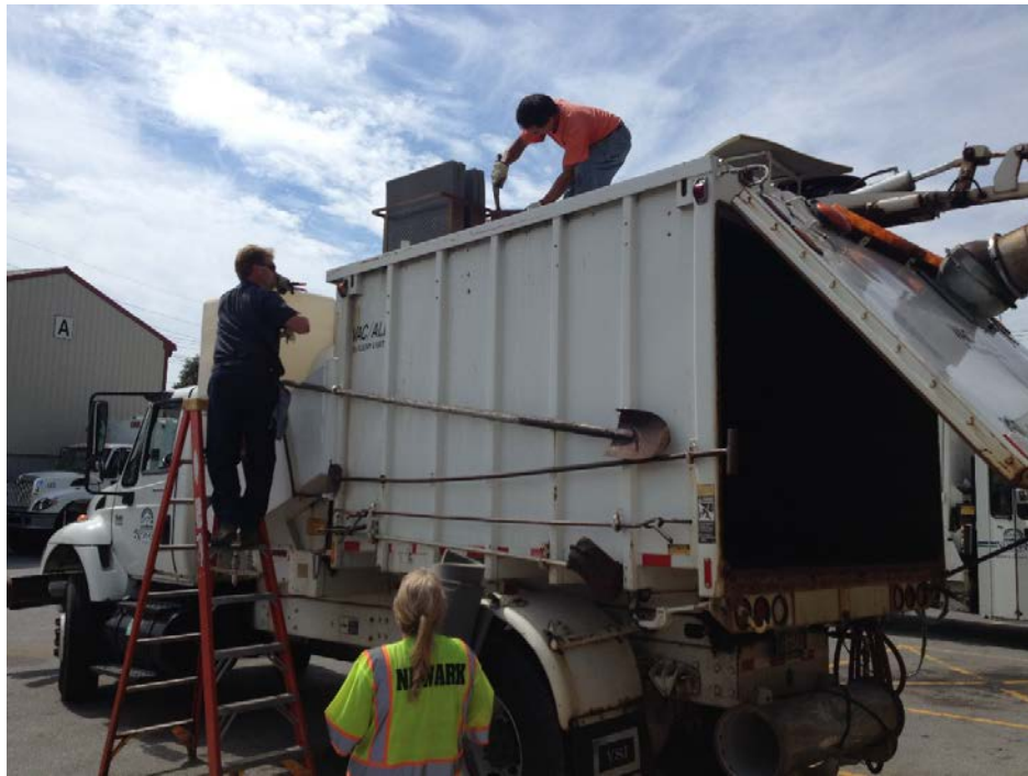
Figure 2: Screen repair of Catch Basin Truck #250
